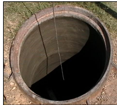
After - structural restoration.
